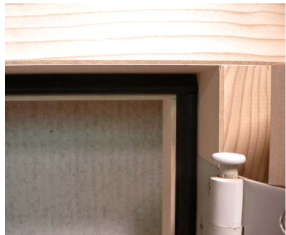
A properly prepared opening and the proper installation of gasketing (above) are critical to the field performance of an acoustical door.
